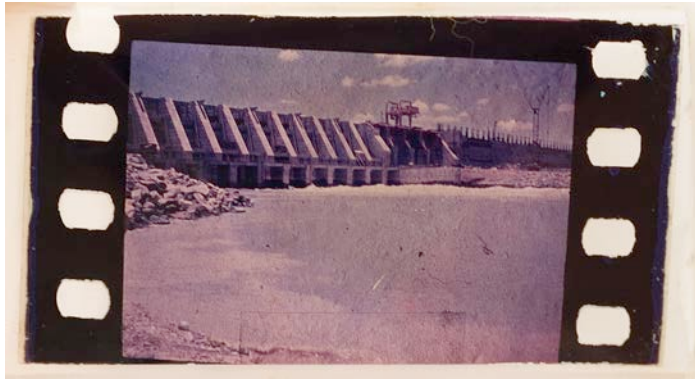
FIGURE 4.2. Sobradinho dam works (s.d.).
