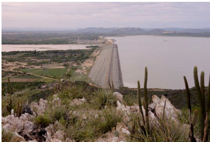
FIGURE 4.3. The Sobradinho dam in May 2015.
